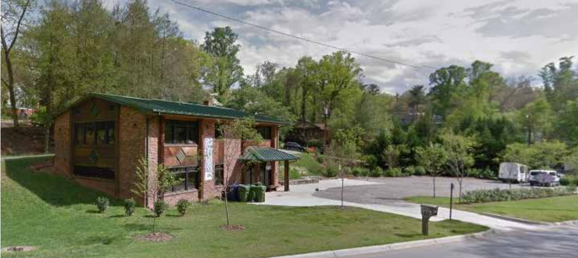
Hanger Hall School for Girls is located on WT Weaver Boulevard in the 5 Points neighborhood, across the street from Glenn's Creek Greenway..
